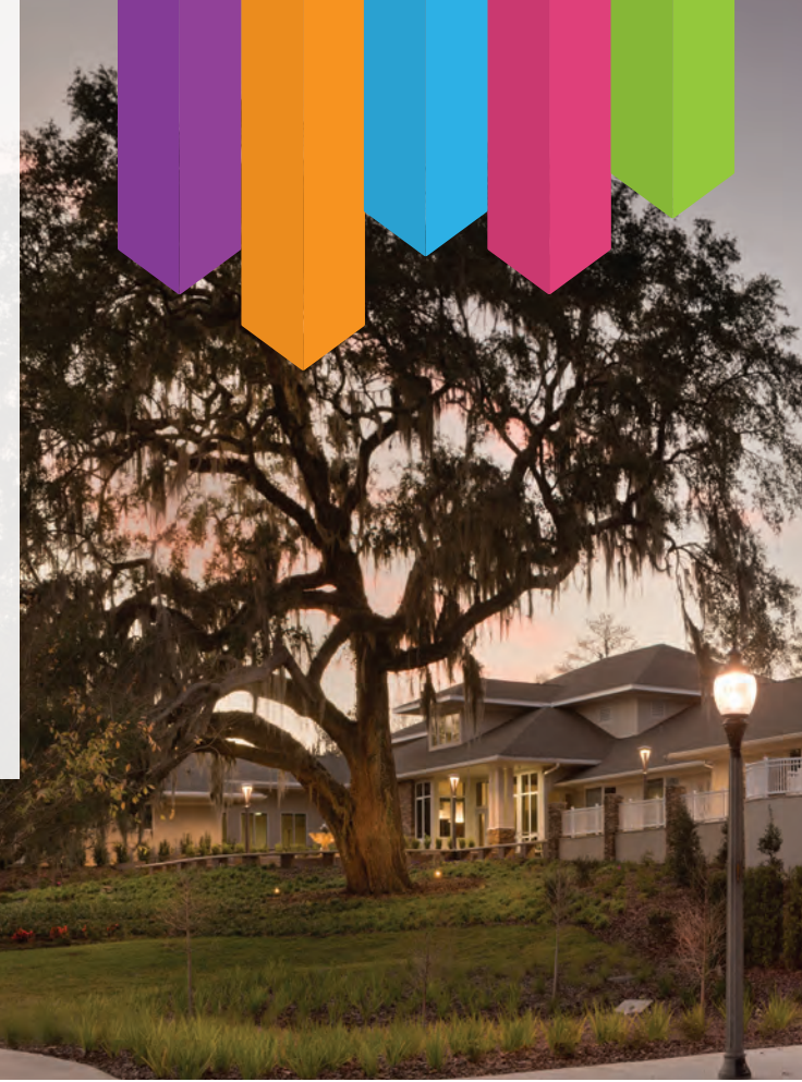
The newly expanded E.T. York Care Center in Gainesville
